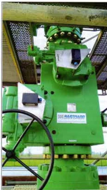
Fig. 5 Block-design of integrated cross, wing valve and top valve
