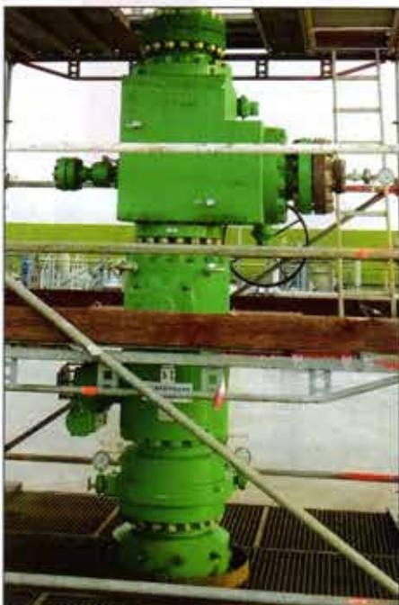
Fig. 6 Gas storage wellhead with integrated valves
