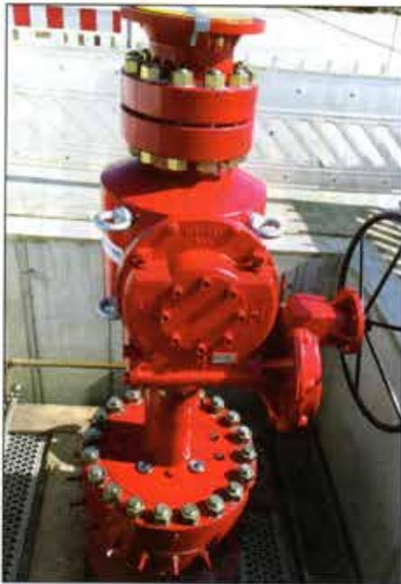
Fig. 2 Geothermal wellhead with eccentric hanger
