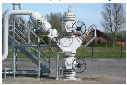
Reliable combination: Hartmann gas wellhead with gas-tight, metallic sealing ball valves in Jemgum, Germany.
