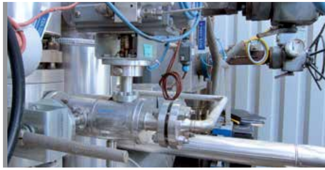
Absolutely gastight: the true metal to metal sealing ball valves by Hartmann Valves made of Inconel 625® (solid material)
