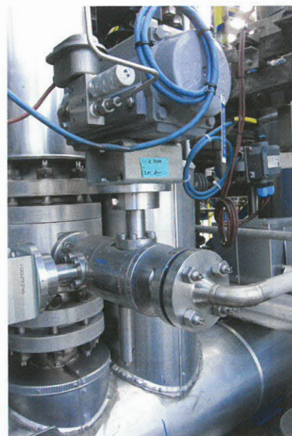
The four reactors of the POX-gasification plant at Yara Brunsbüttel with their gastight and metal-to-metal sealing ball valves – a customized Hartmann design for high temperatures, steam and pure oxygen.
