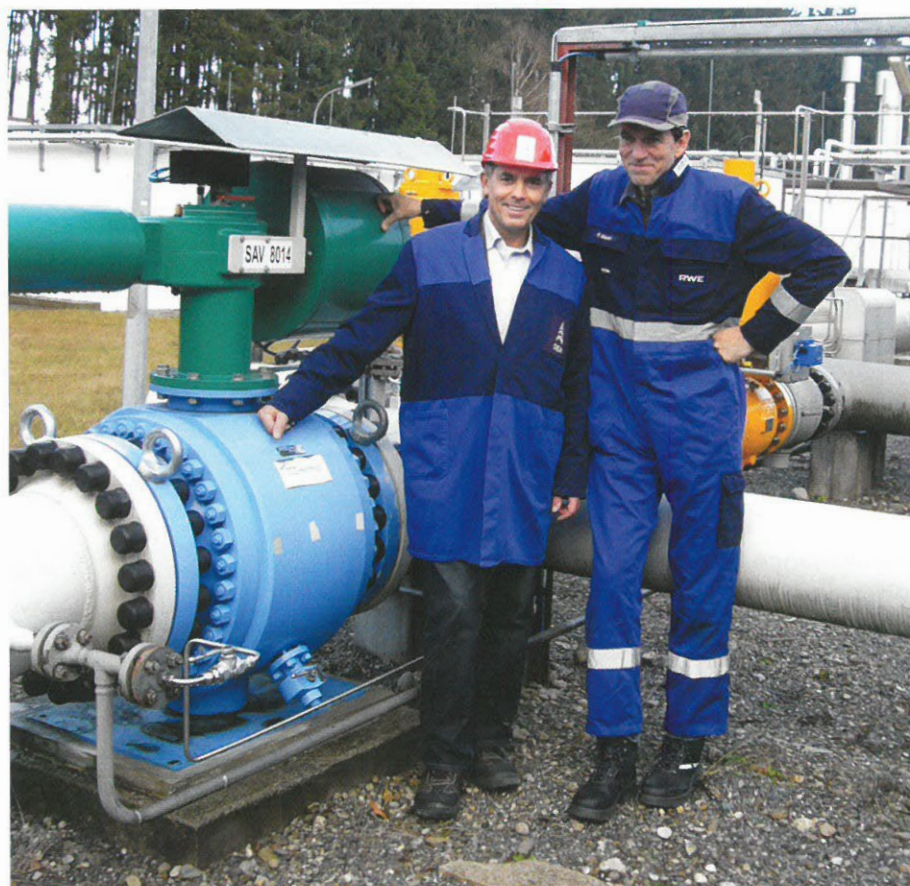
Plant Manager and Hartmann Manager at the DEA Gas storage facility where 800 Hartmann metal-to-metal sealing ball valves ensure high safety requirements.
