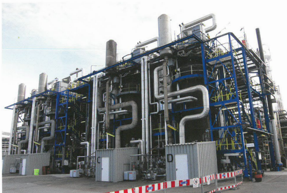
The four reactors of the POX-gasification plant at Yara Brunsbüttel with their gastight and metal-to-metal sealing ball valves – a customized Hartmann design for high temperatures, steam and pure oxygen.
