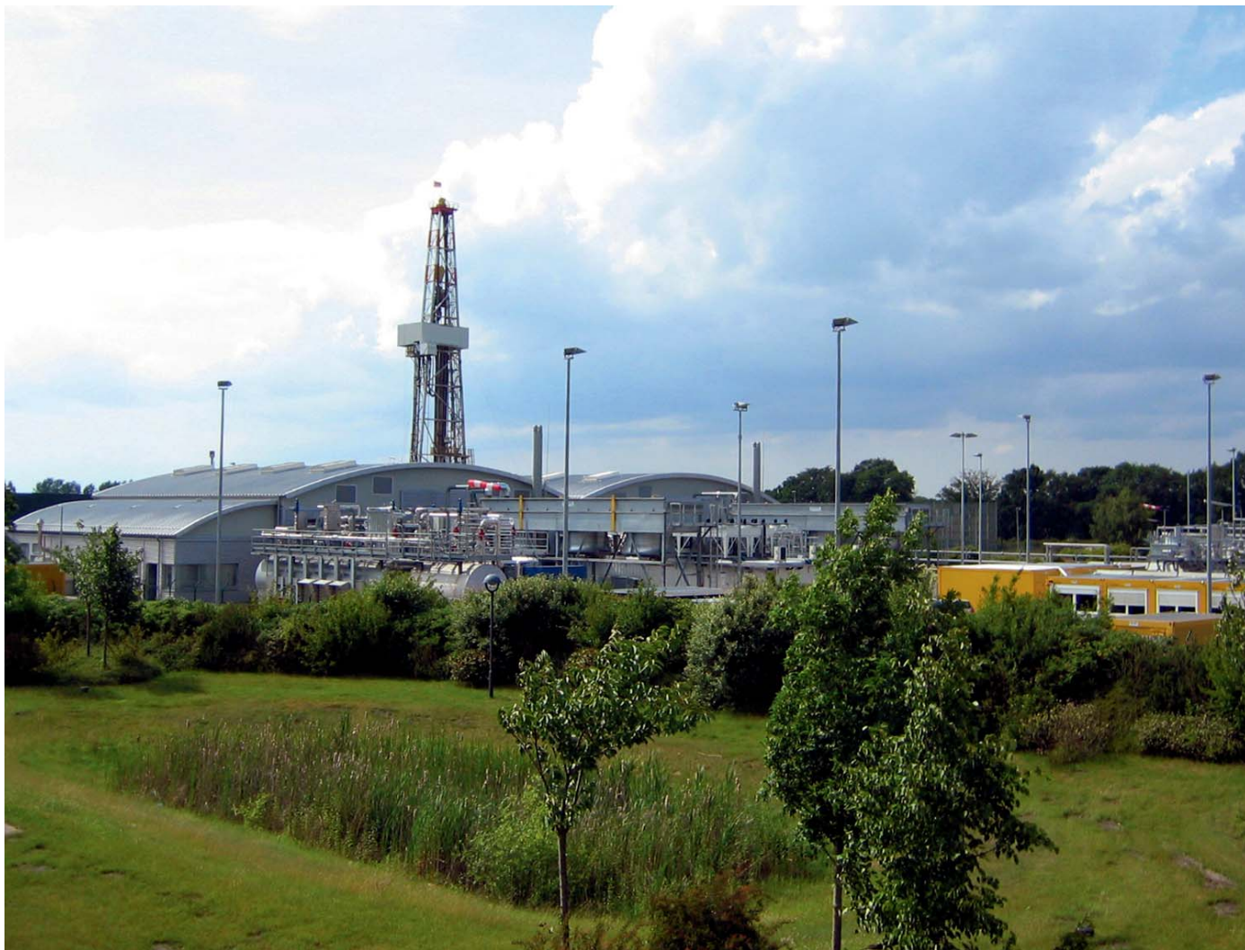
The central gas drying plant of DEA Deutsche Erdoel AG in Völkersen (Germany).
