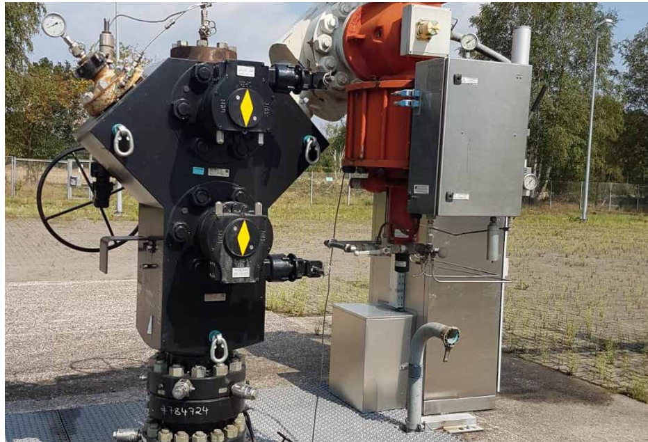
Successful changeover: The Xmas tree with ball valves and quick-closing valve is deployed virtually maintenance-free in gas production.
