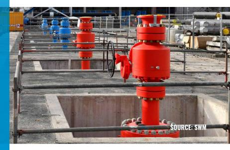
As a leading wellhead supplier in German deep geothermal energy, Hartmann Valves is supporting Stadtwerke München (SWM) by implementing their district heating vision: Munich will be Germany´s first major city where district heating is produced 100% from renewable energies, especially from geothermal applications by the year 2040.
