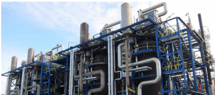
The four reactors of the POX-gasification plant at Yara Brunsbüttel
